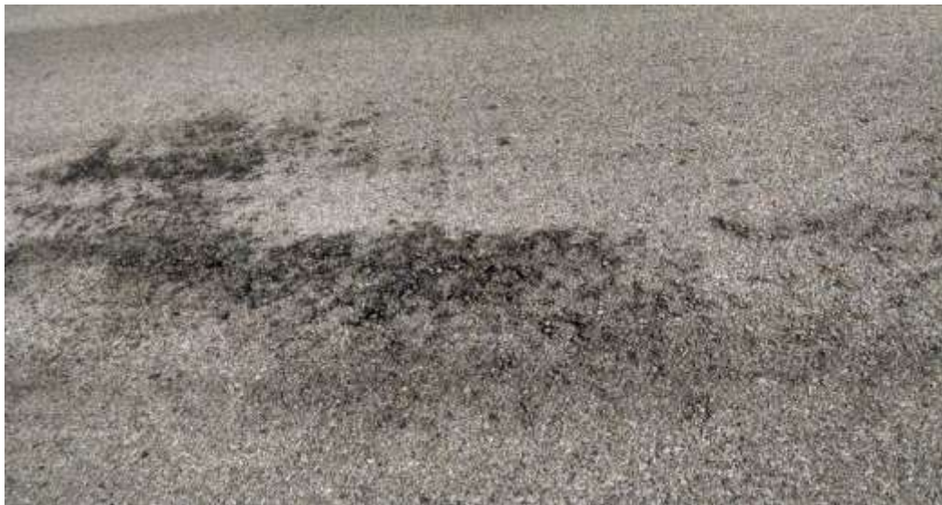
Hydraulic leakage on the runway surface
