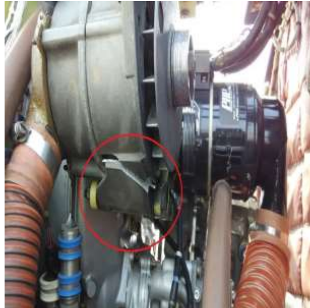
Generator casing rupture due impact
